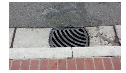
Step 5 - Insert cover into frame immediately. Wait additional 5 minutes before placing in traffic loading.
