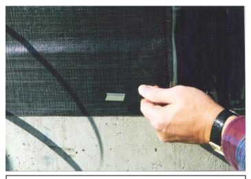
5. Bend the end of the band back and under the clip.
