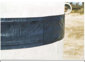
10. Place closing flap over the exposed straps to complete the installation.
