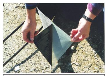
2. Remove a portion of the protective plastic fil from the back side if the seal wrap to expose mastic.
