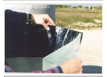
9. Remove the protective plastic film from the back of the closing flap.
