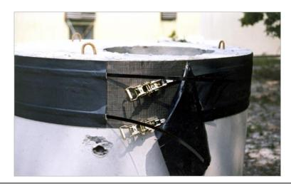
1. Sweep or brush external portion of the joint to insure foreign materials do not interfere with the direct contact between the mastic sealer and the joint to be sealed. Align the collar directly over the joint to where the straps close over the top of the pipe. Remove the protective plastic film, exposing the mastic side to the joint. Wrap the exposed mastic around the joint.
