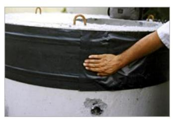
3. Remove protective film from the closing flap to cover the two tensioning ratchets and straps, completing joint. Cretex Wrap equipped with high tensioning ratchets provides a positive seal on box, arch, elliptical and round pipe.
