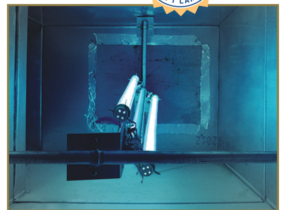
3. OEO System in duct
