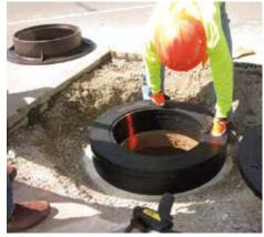
Place the Angle Ring onto the Finish Ring with the adhesive facing down, making sure to align with any previously applied marks.
