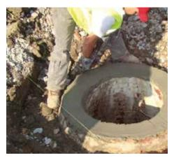
If the surface on top of the manhole is too damaged, rough or irregular, place a ½" thick bed of non-shrink mortar or grout on the surface and rough in.
